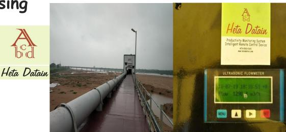
For a 70 KM long Pipeline designed to carry 1500 CUM/hr of water, only 750 CUM/hr water reached the source. The air was to improve the Pumping Efficiency, and locate the water leakage or pilferage. The pipeline was mostly underground, and passing through forest aera.
